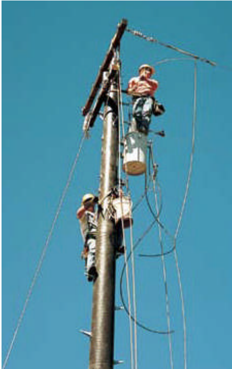
Figure 10 A Shakespeare composite utility pole [16]. Photo by Shakespeare.
