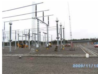
Construction works in Finnböle 400 kV AC switchgear, November 2009
