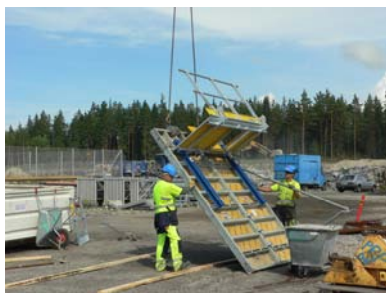
Setting up the casting mould at Rauma Summer 2010
