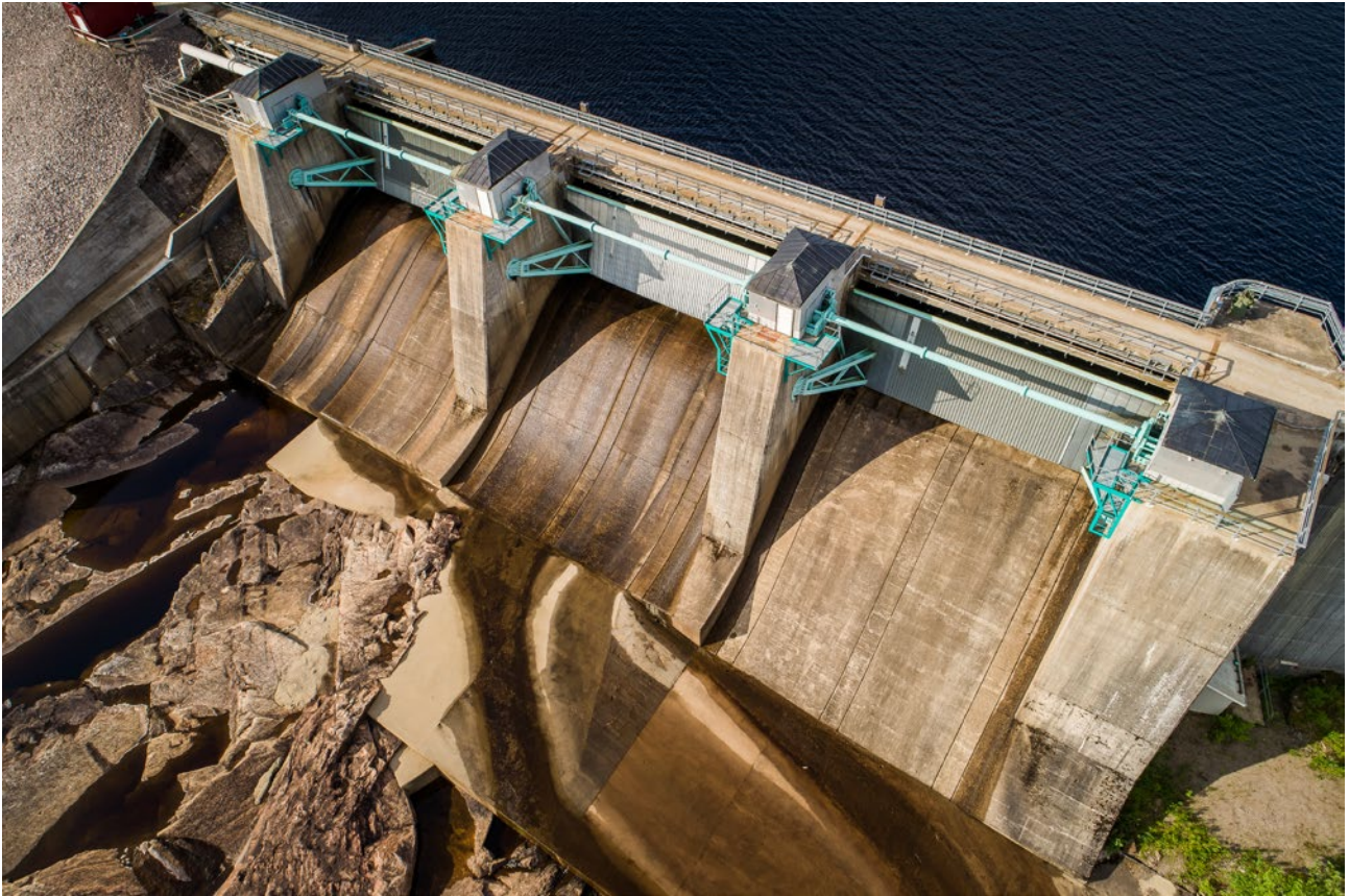
Overview of the discharge structure with three segmented gates at the Krokströmmen dam. Photo: Svenska kraftnät.
