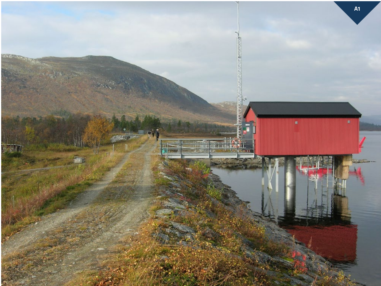
The Burvattnet dam, completed in 1943, is an embankment dam with a wooden diaphragm. The dam is situated in located in roadless land and was recently refurbished. Photo: Vattenregleringsföretagen.
