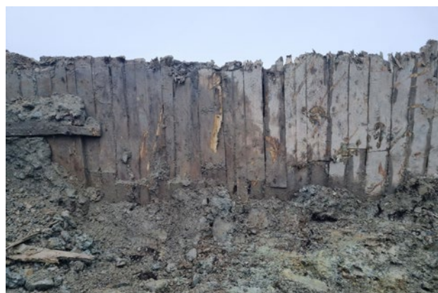
Wooden diaphragm wall at Burvatten dam, during original construction and excavation in 2022. Photo: Tina Pålhlstorp.
