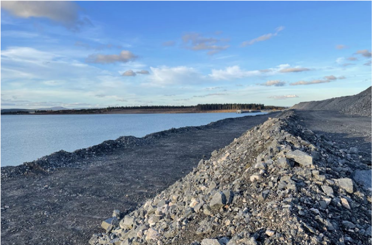
Detail, buttress on dam E-F, Clarification pond to the left, TSF to the right (2021).
