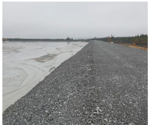
Figure 3. Dam crest and upstream area with the tailings overflow at VSD.
