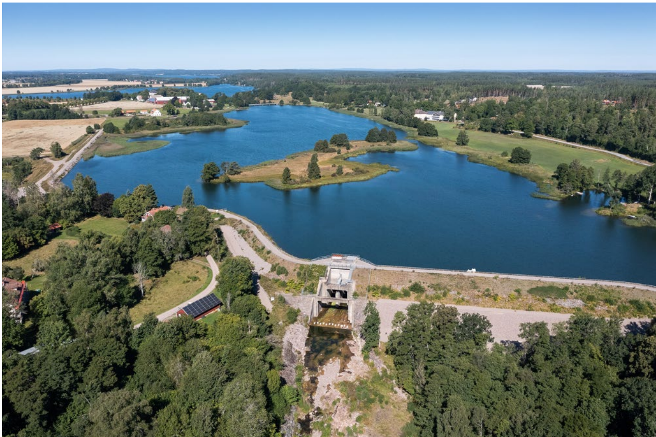
The Malfors dam, an early successful example of a high Swedish embankment diaphragm dam, was built in 1934 and is 15 meters high. The dam features an inclined concrete diaphragm with surrounding clay mixed with sand. Photo: Svenska kraftnät.
