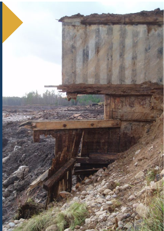
Dam failure in Hästberga Dam 2010. Photo: Maria Bartsch.
