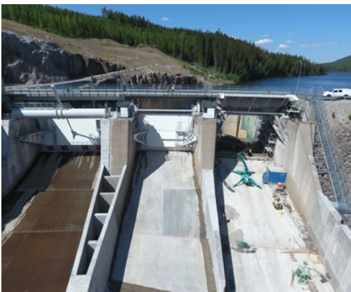
Surface spillway with radial gates.
