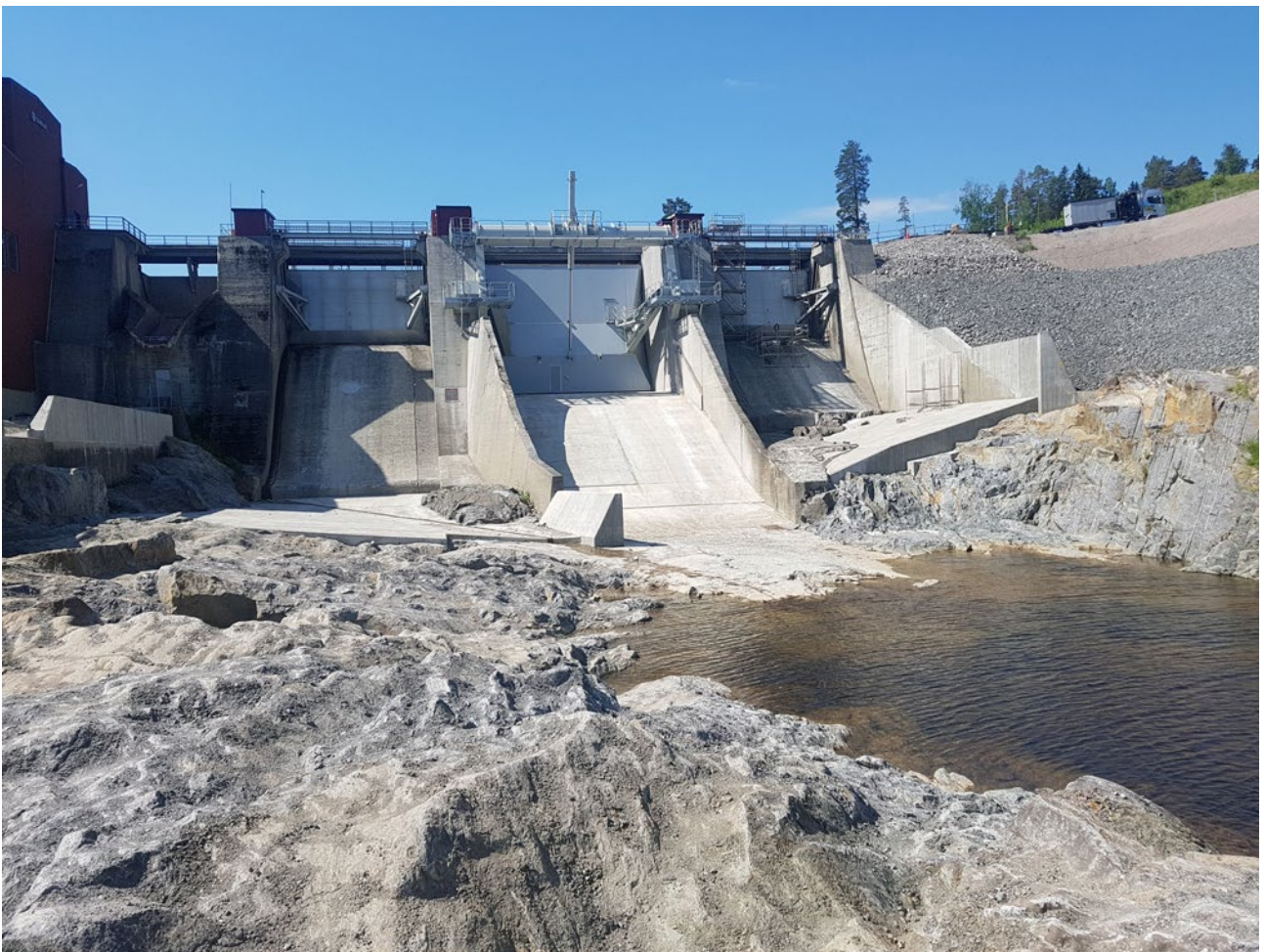
Rebuilt spillway 2.
