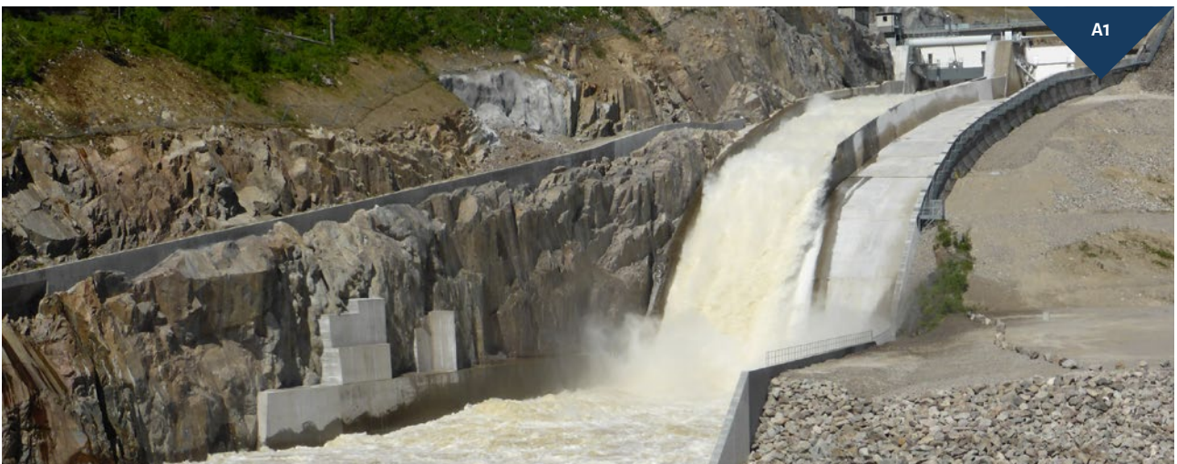
The Höljes dam is an example of a large embankment dam with a discharge structure on one of the shores. The water is discharged via a stilling basin. Photo: Fortum.
