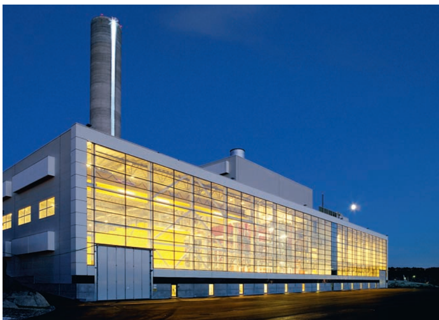
The Rya combined heat and power plant came on line in Göteborg at the turn of the year 2006/2007. The plant has a capacity of 260 MW of electricity and 290 MW of heat and is today the largest single consumer of natural gas in Sweden.
